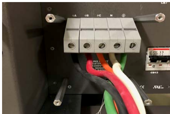
Figure 1-1. AC Line Cord Installation
