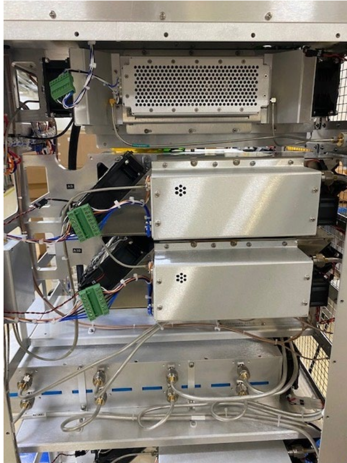
Figure 4-5. 2500A225C, Right Side, Modules A9-A12
