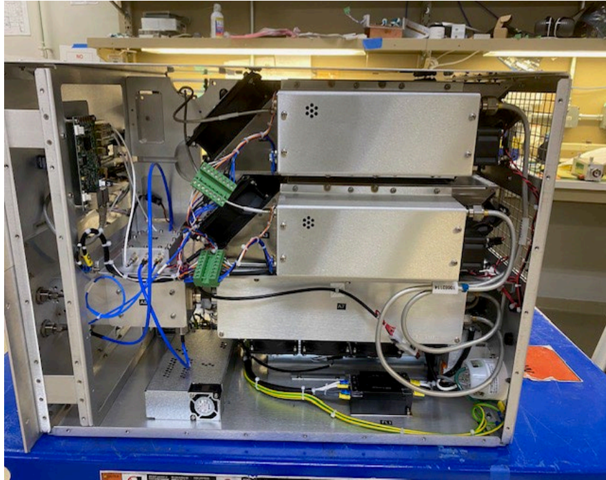
Figure 4-5. 1200A225B, Right Side, Modules A3-A5.
